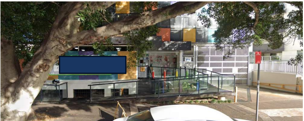
Figure 4-2 Higher Density Example of Development of a Flood Affected Multi-Storey Building with Elevated Ground Floors, Elevated Basement Carpark Entry and Flood Storage under Suspended Ground Floor
