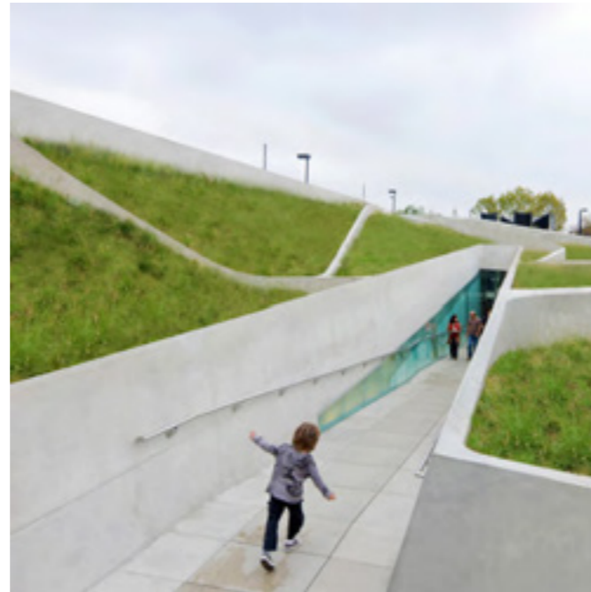
2. Building entrances sliced into incline
