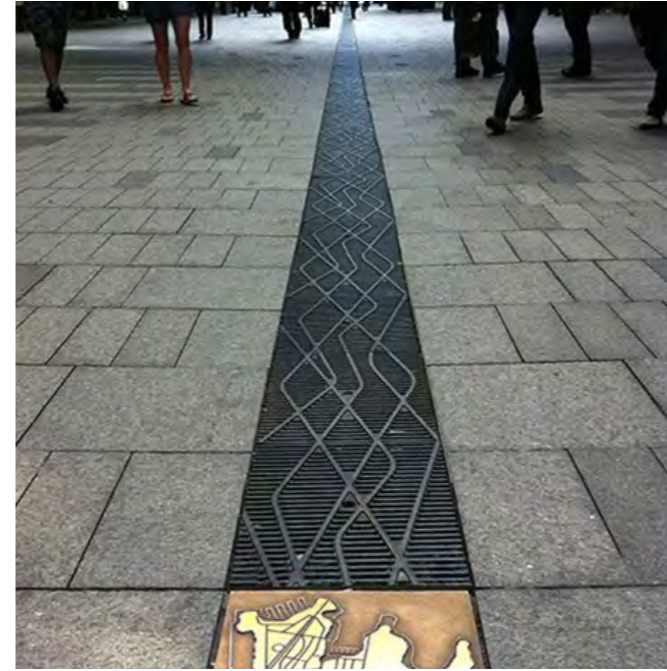
3. Linear water channel
