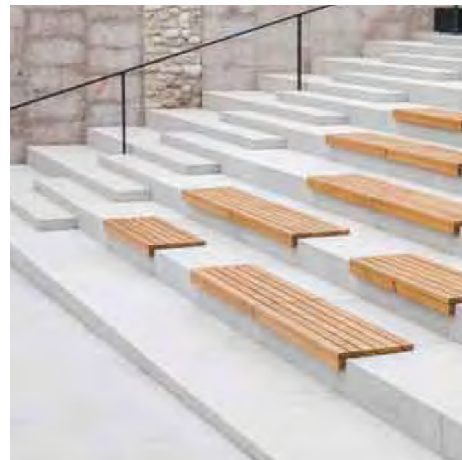
6. Concrete walls and seating edges
