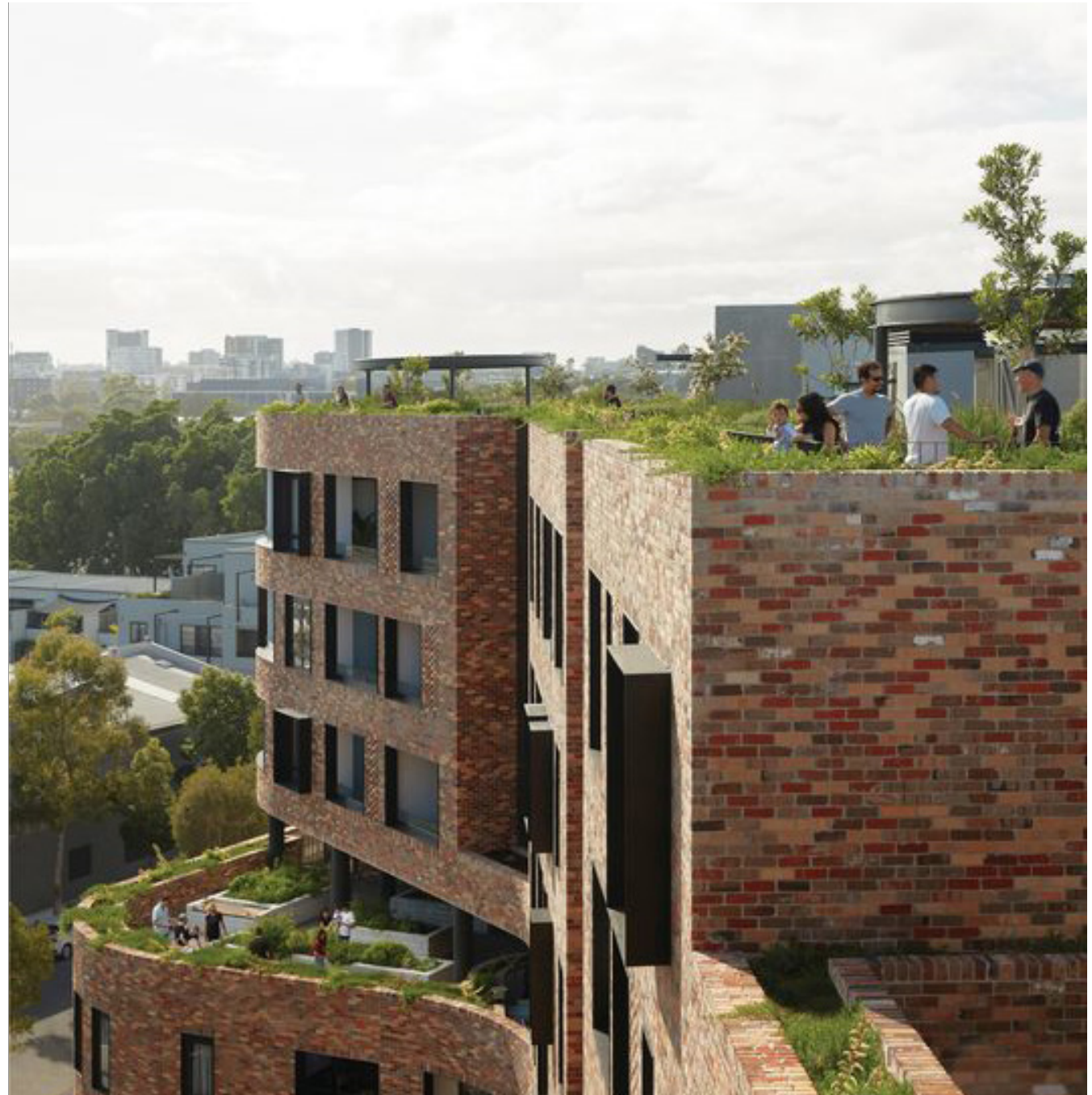
Figure 33. Podium exposure to enhance solar access, Arcadia.
