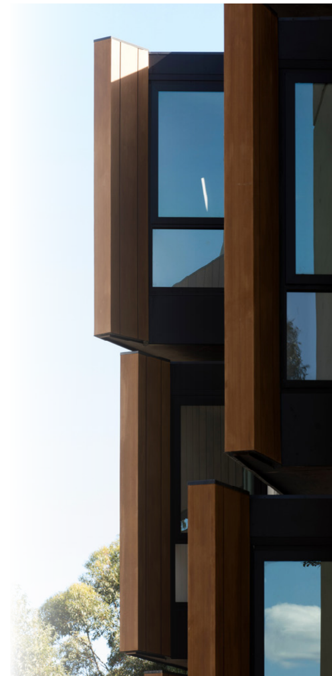
Figure 35. Shoutridge, Lindfield NSW, Architectus (Source: Brett Boardman)
