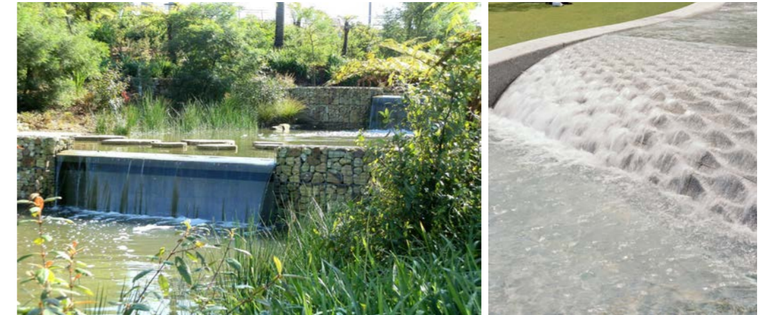
AN EXPANDED UPPER POND AND RECONFIGURED CHANNEL WITH CASCADES TO IMPROVE WATER HEALTH
