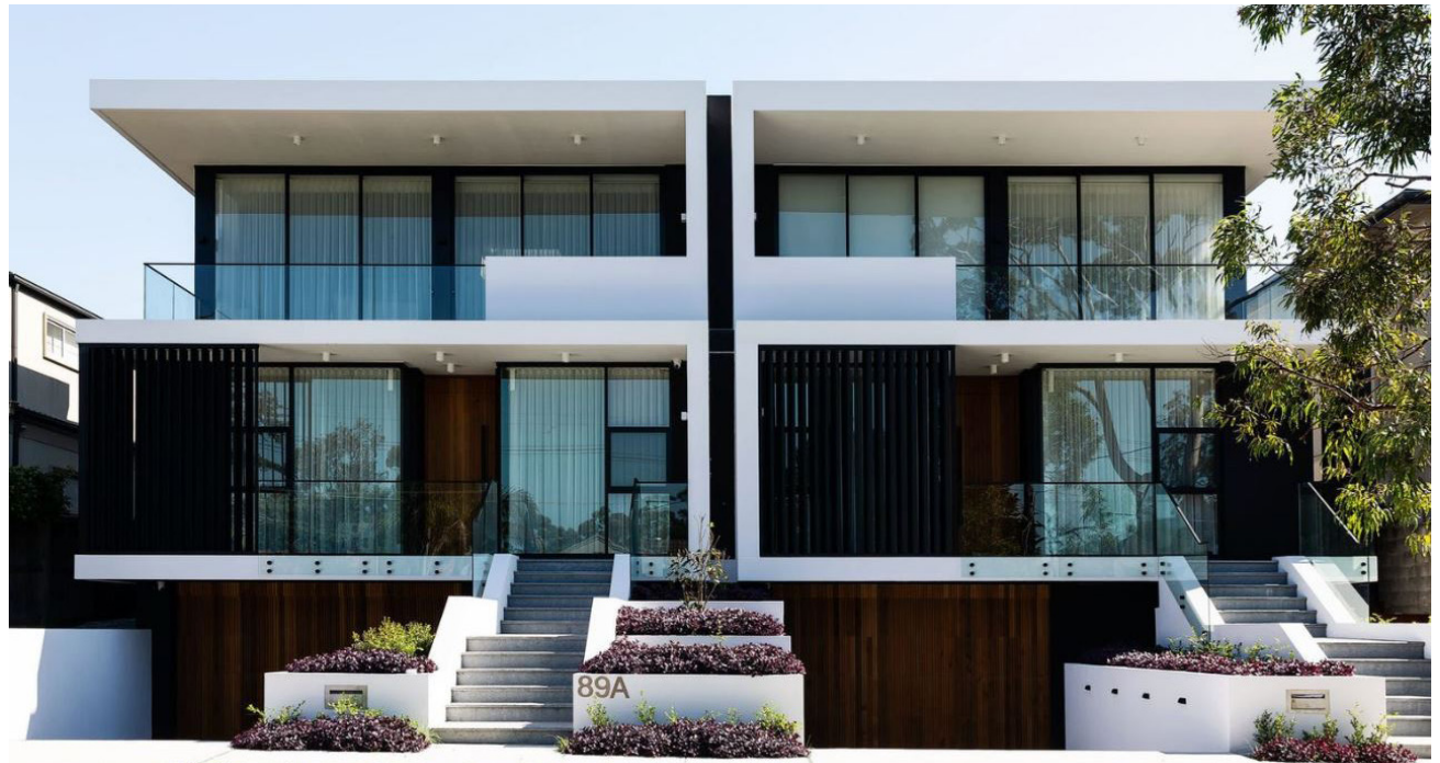
Basement parking in low-rise housing (Sydney, NSW).
