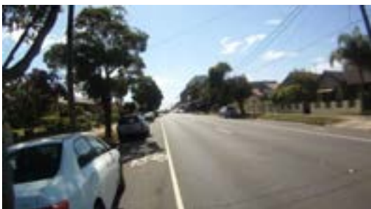
Figure 5.9: Bike Lane in the Door Zone
