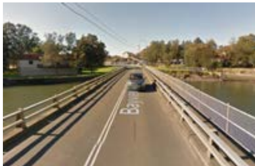
Figure 12.16: Narrow bridge and footpath (looking east)
