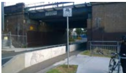
Figure 12.9: Existing Conditions at the Charles Street Underpass
