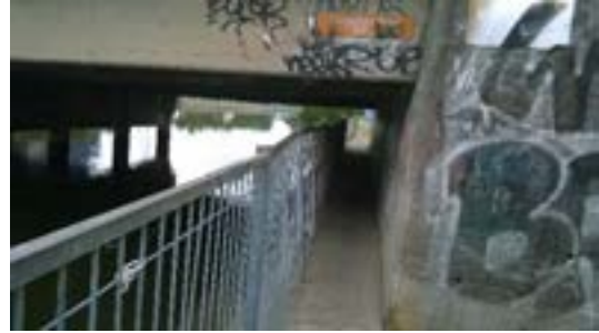
Figure 12.2: Existing Conditions at the Cooks River Underpass
