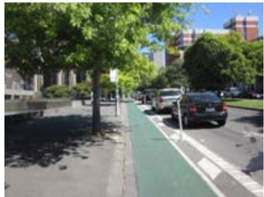
Figure 7.8: Albert Street, Melbourne - low-cost median
