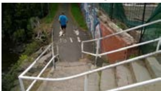
Figure 12.6: Existing Steps at the Homer Street / Illawarra Road Bridge
