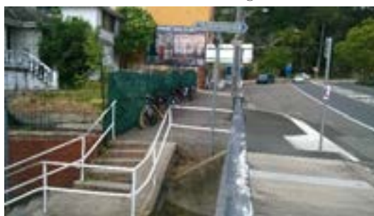
Figure 12.7: Existing Steps at the Homer Street / Illawarra Road Bridge
