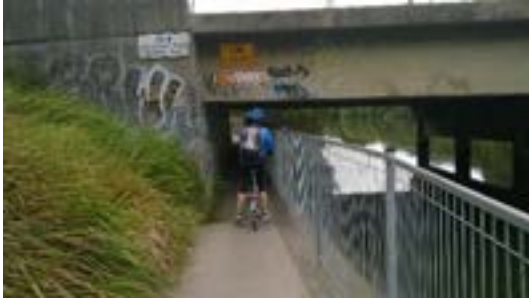
Figure 12.1: Existing Conditions at the Cooks River Underpass
