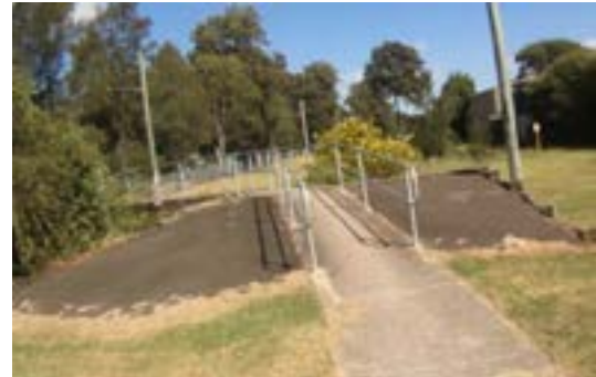
Figure 12.13: Narrow, pedestrian-only bridge
