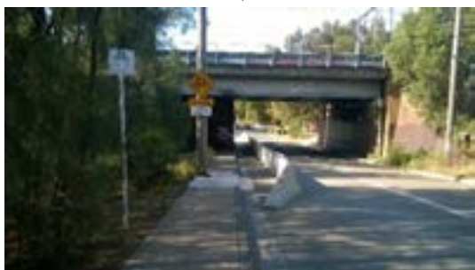
Figure 12.8: Existing Conditions at the Charles Street Underpass
