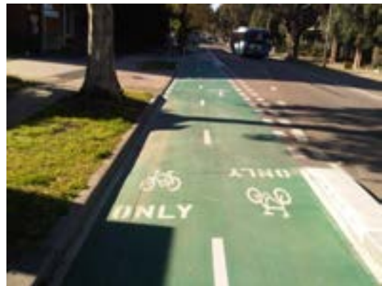
Figure 7.4: Bourke Road, Sydney - in-situ concrete median
