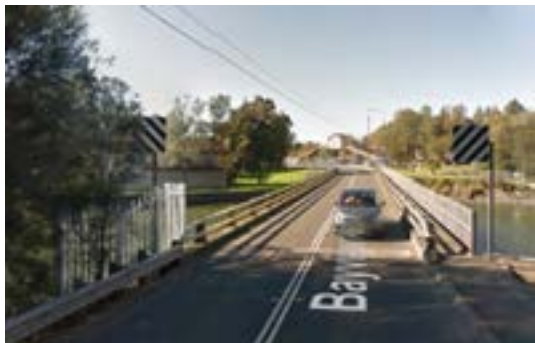
Figure 12.15: Narrow bridge and footpath (looking east)
