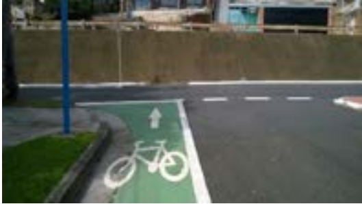
Figure 5.3: On-Road Bicycle Approach Treatment (Bankside Ave)
