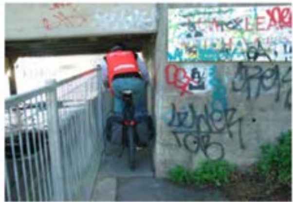
Looking North at Canterbury Road Bridge
