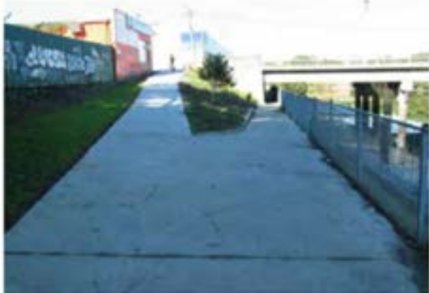
Looking South at Canterbury Road Bridge
