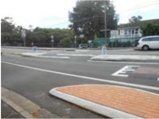
Figure 5.34: Retro-fitted Staged Crossing
