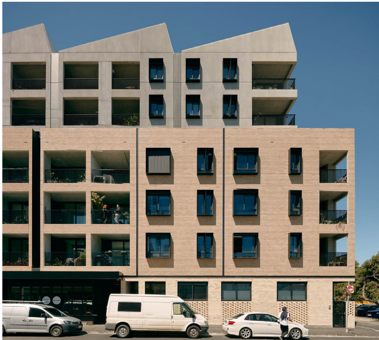
A four storey street wall with upper storey setbacks provides a reduced building scale appropriate for the street and local context, Breese Street, Brunswick, VIC, by Breathe Architects (Source: Tom Ross)
