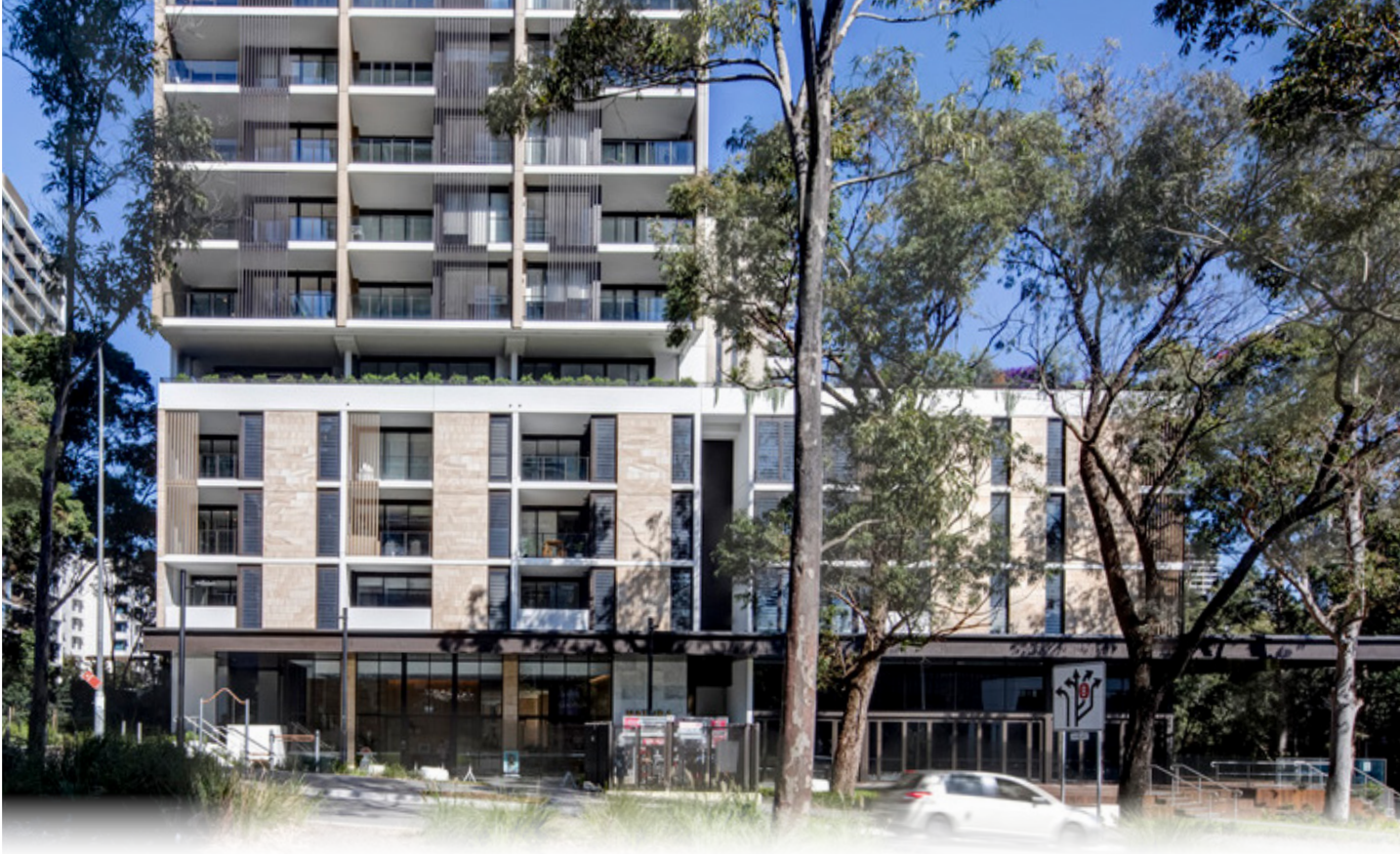
Macquarie Park, NSW, by Architectus (Source: Brett Boardman)
