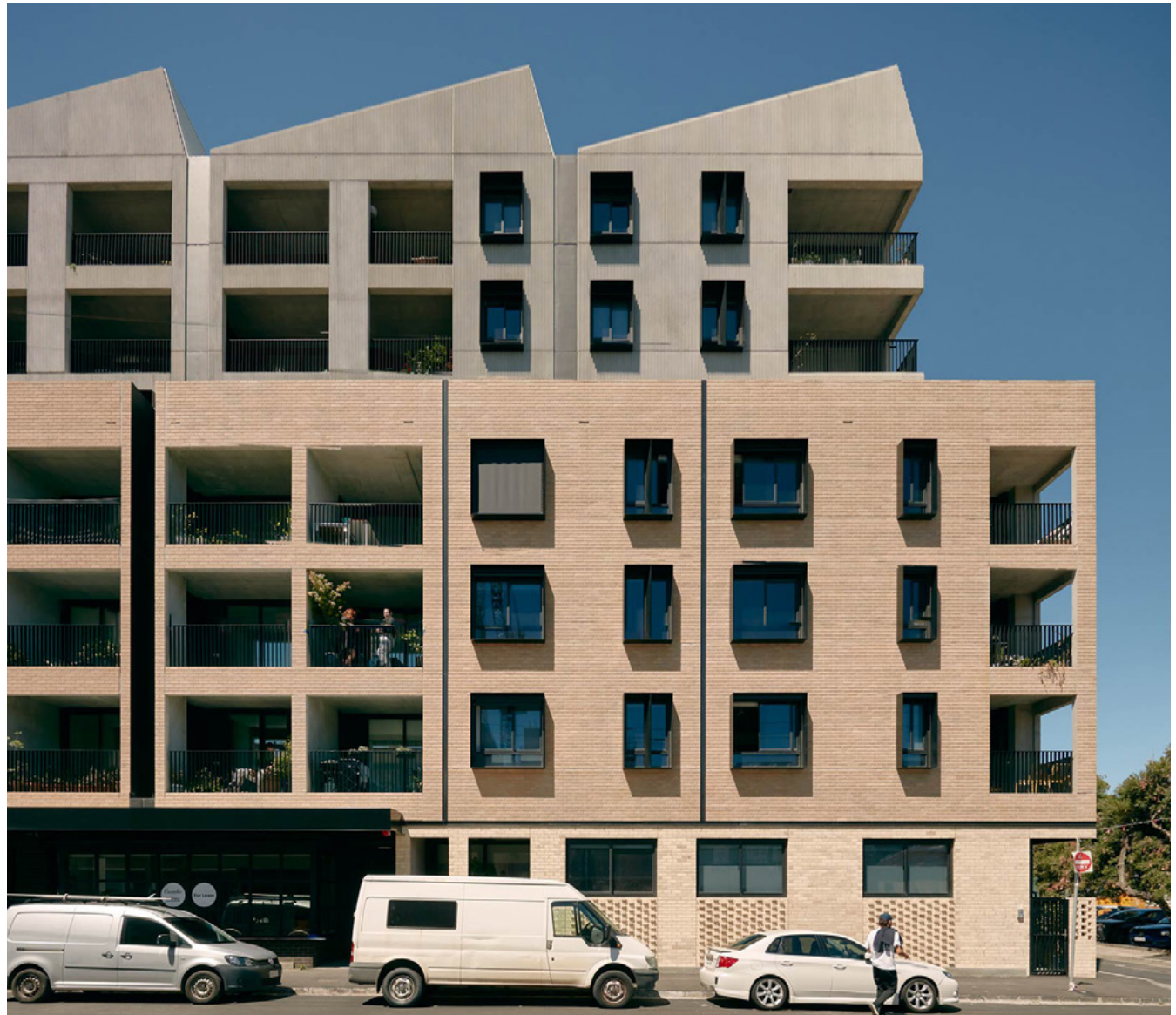
A four storey street wall with upper storey setbacks provides a reduced building scale appropriate for the street and local context, Breese Street, Brunswick, VIC, by Breathe Architects (Source: Tom Ross)
