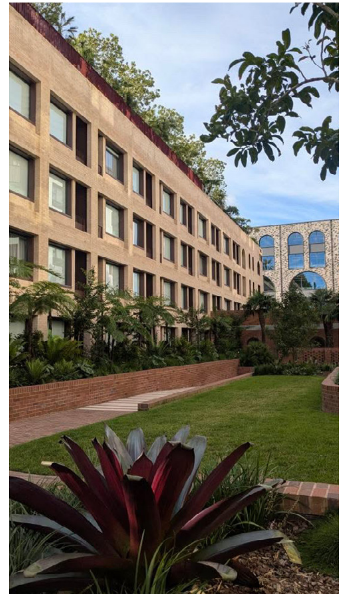
Podium with grass and landscaping, Surry Hills Village, NSW by SJB (Source: Architectus)
