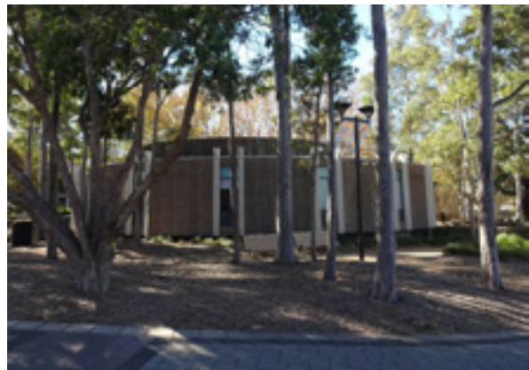
Figure 18 – View towards side elevation of Council Chambers.
