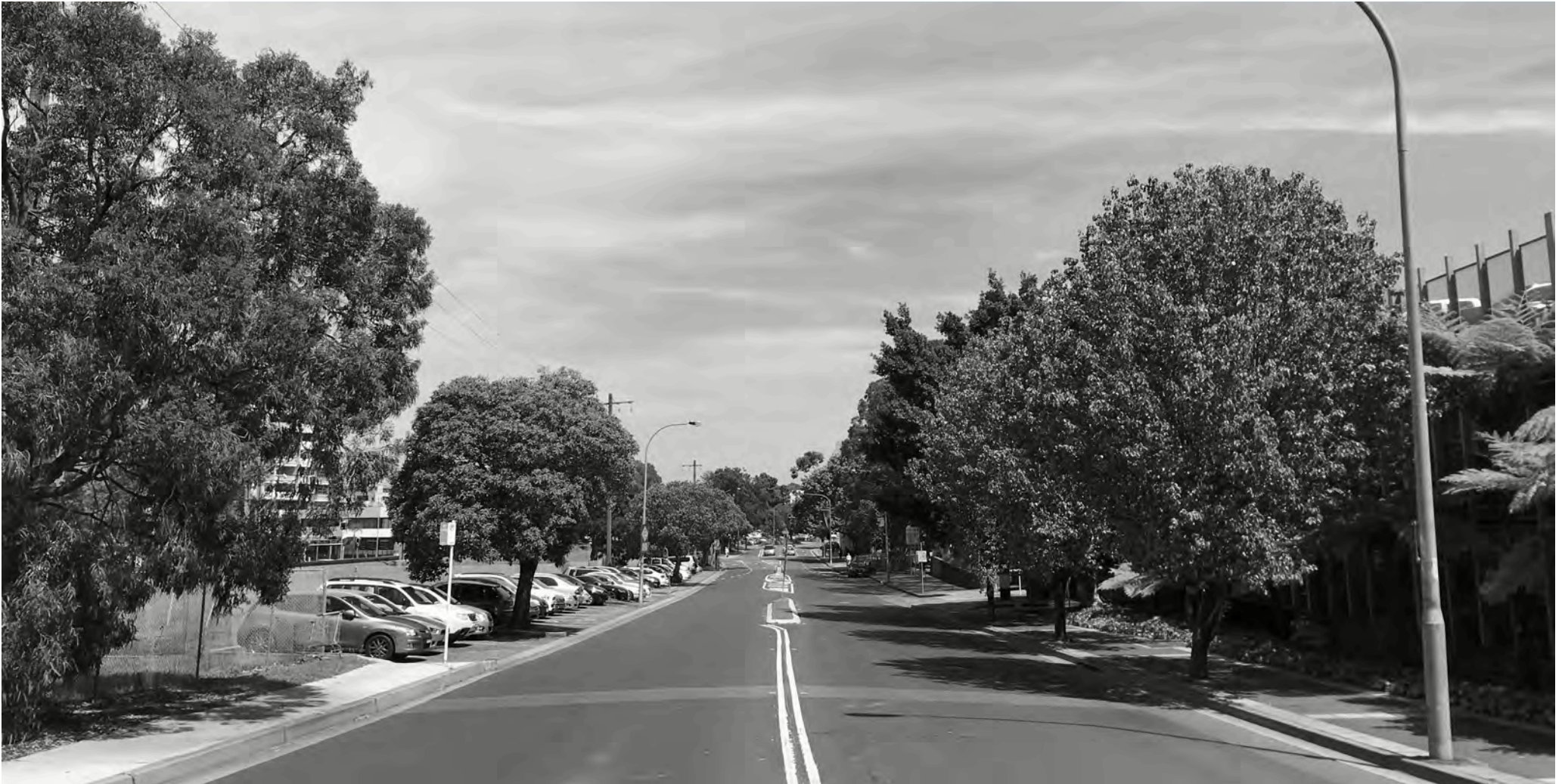
Existing View (looking West)
