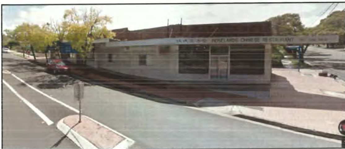
Photograph 1: 89-95 Karne Street North (looking north-east)
