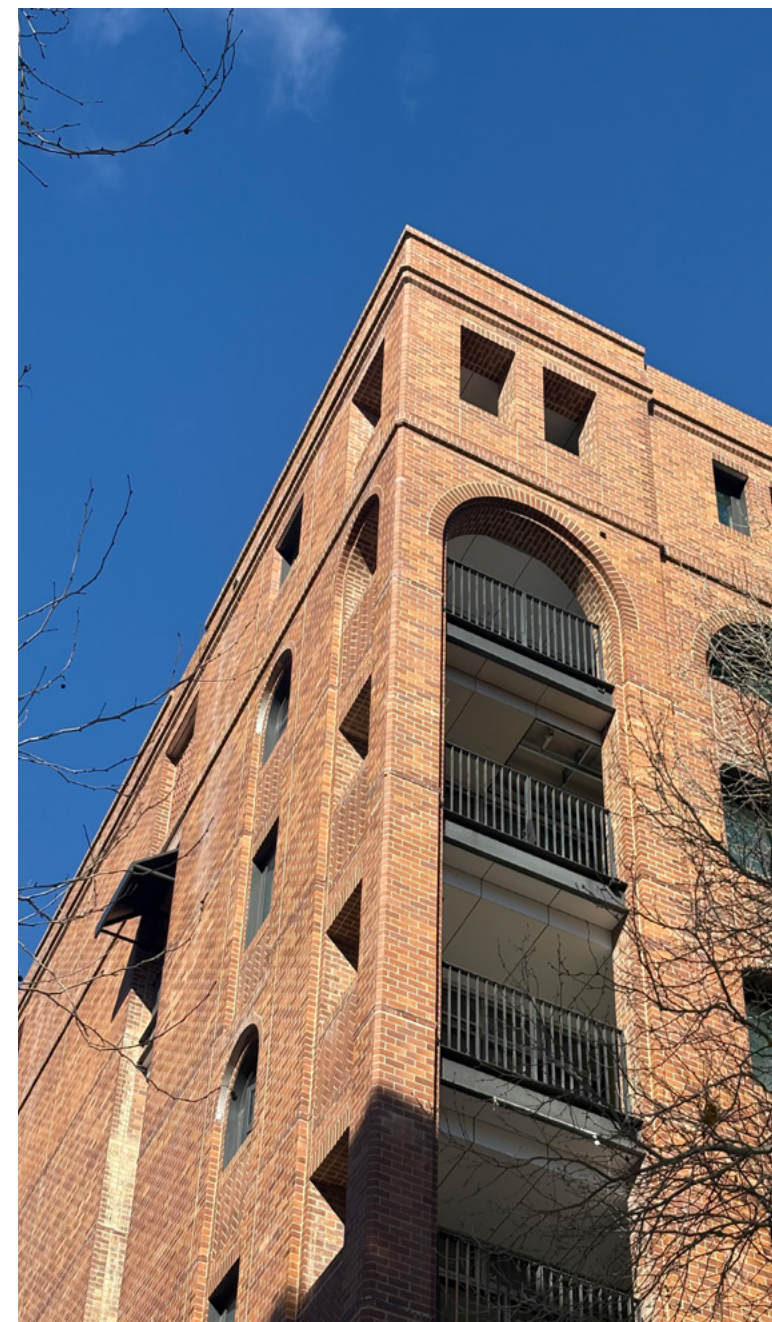
Group GSA LAHC, Glebe NSW (Source: Glyde_Bautovich)
