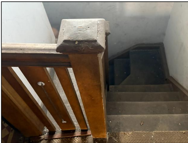
Figure 41: View of staircase including original timber Newell post, balustrade and skirting.
