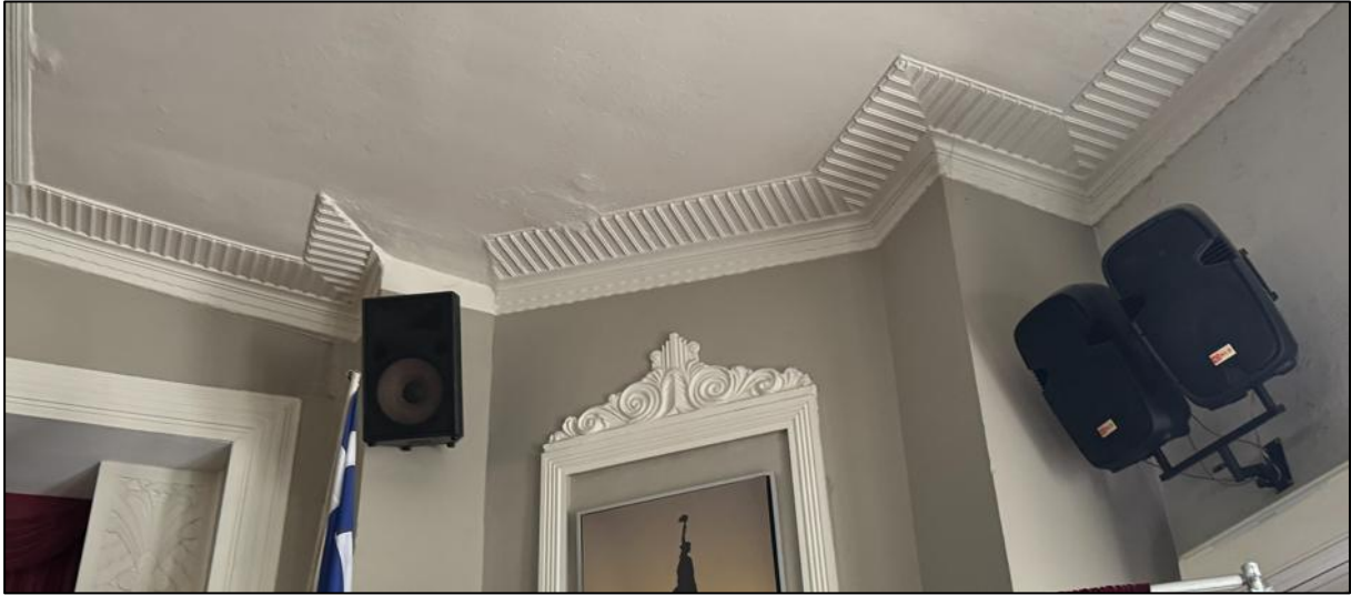
Figure 66: View of upper wall and ceiling of hall space. Modified elements include cut decorative cornice, decorative window elements, audio speakers etc.
