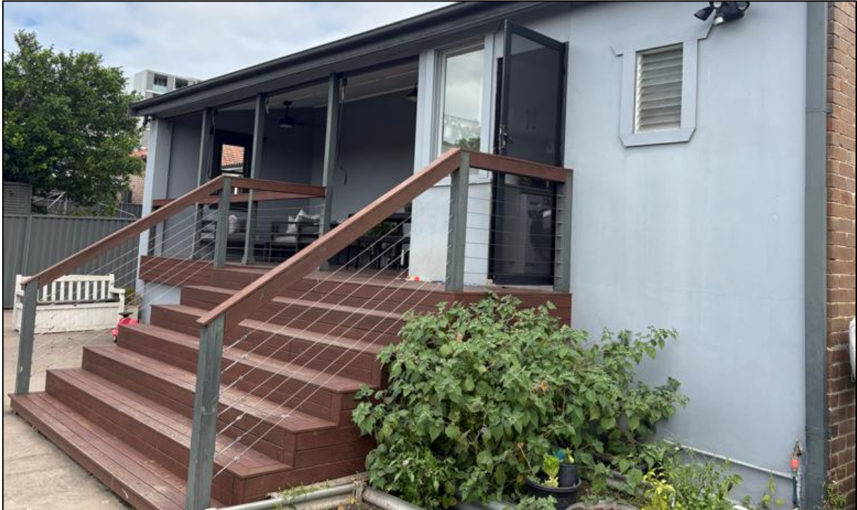
Figure 85: View of rear elevation of the dwelling, showing open deck (former sunroom) with timber stairs leading to backyard.
