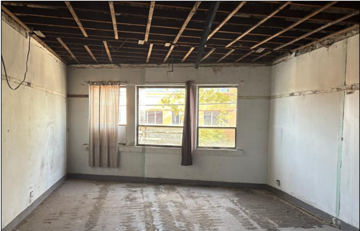
Figure 38: View of the interior first floor of No. 341 Beamish Street.
