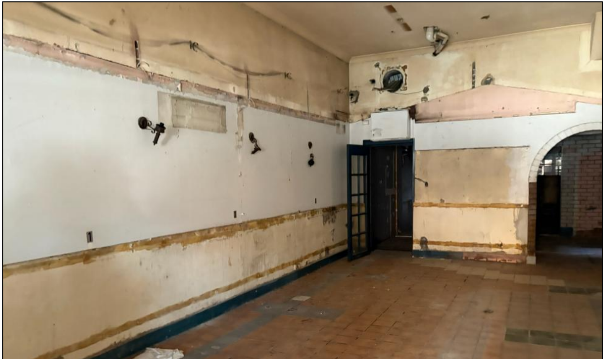
Figure 33: General view of the interior of Shop No. 341.
