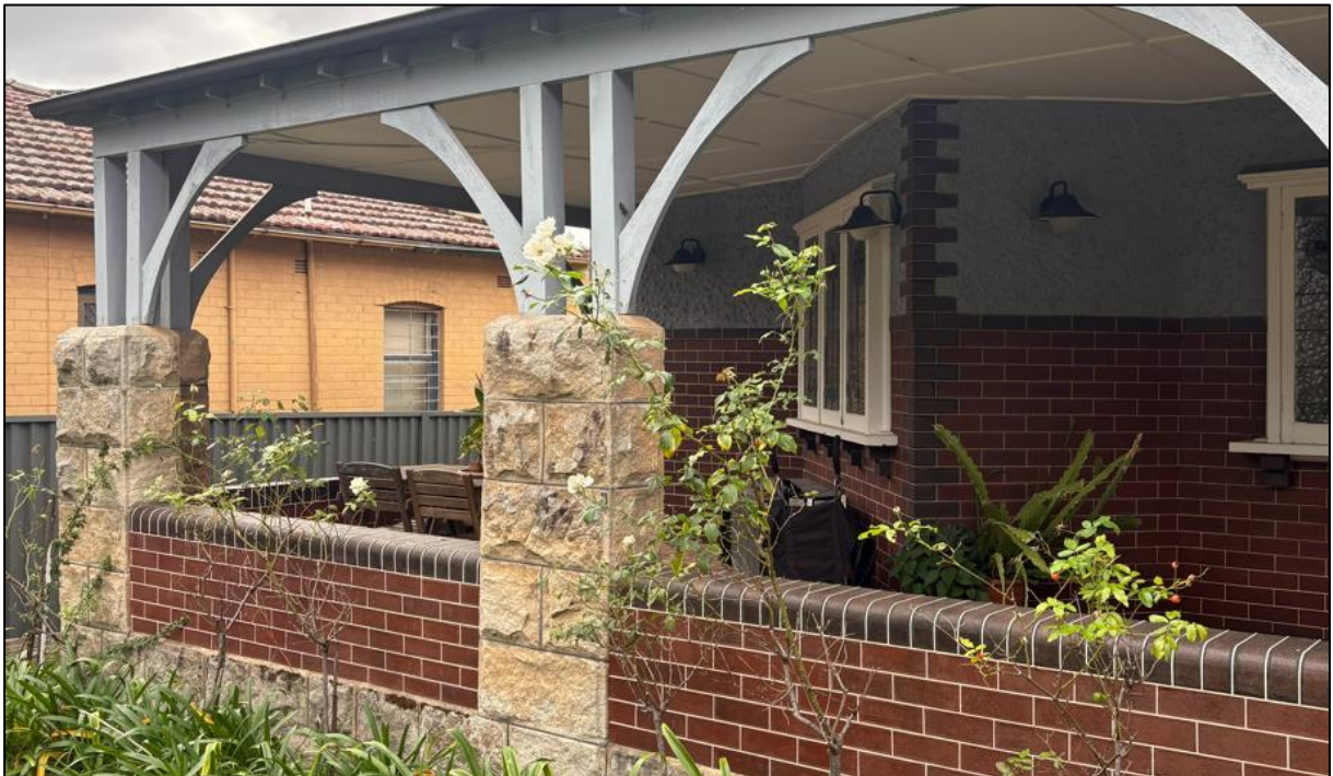
Figure 80: View of front L-shaped verandah and façade of the dwelling.
