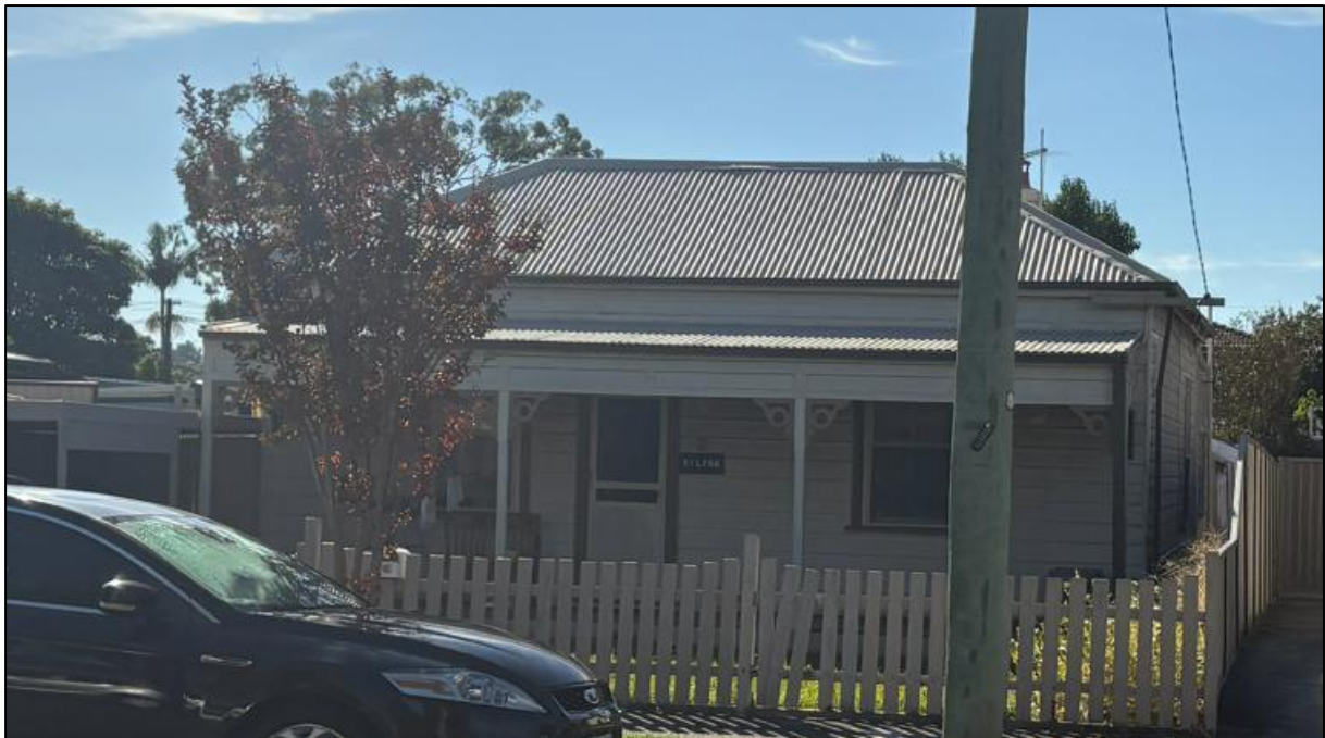
Figure 56: Front elevation of the cottage at 2 Burns Street (identified as 'Wilton').
