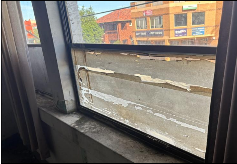
Figure 40: View of first floor windows of No. 341, showing modified architraves.
