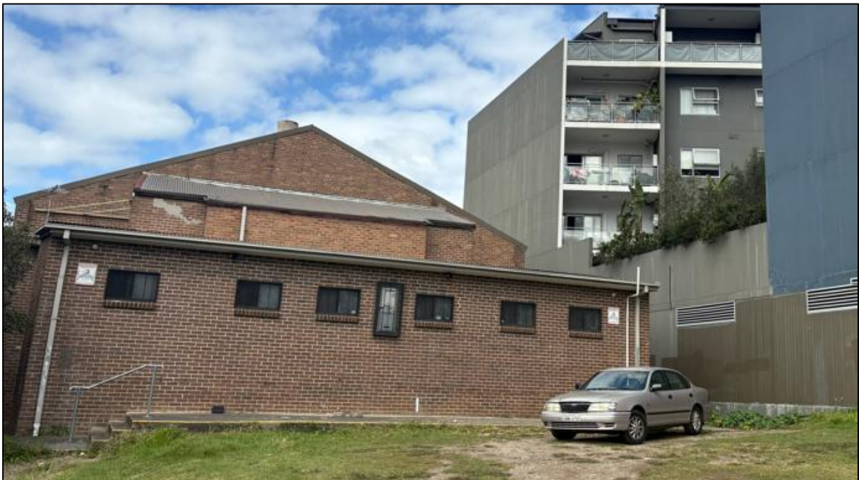
Figure 62: Norther (rear) elevation of the Mytilenian House, featuring c.2000s amenities extension.
