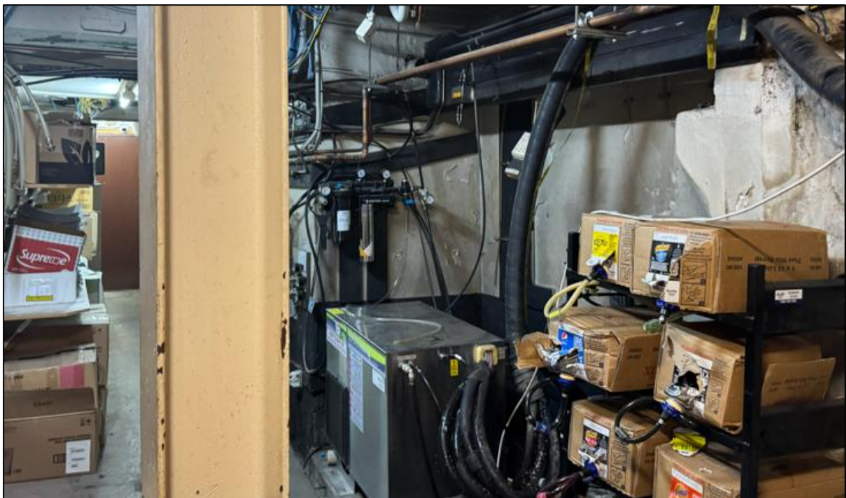
Figure 28: General view of sub-floor basement.
