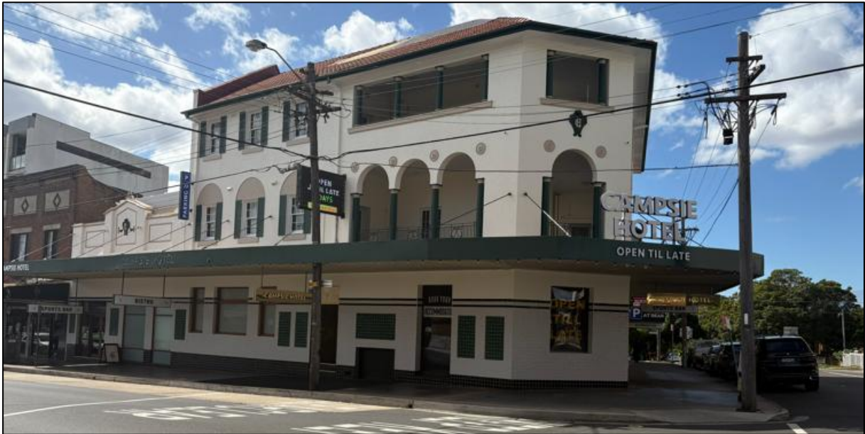
Figure 18: View of the Campsie Hotel, looking east from Beamish Street.
