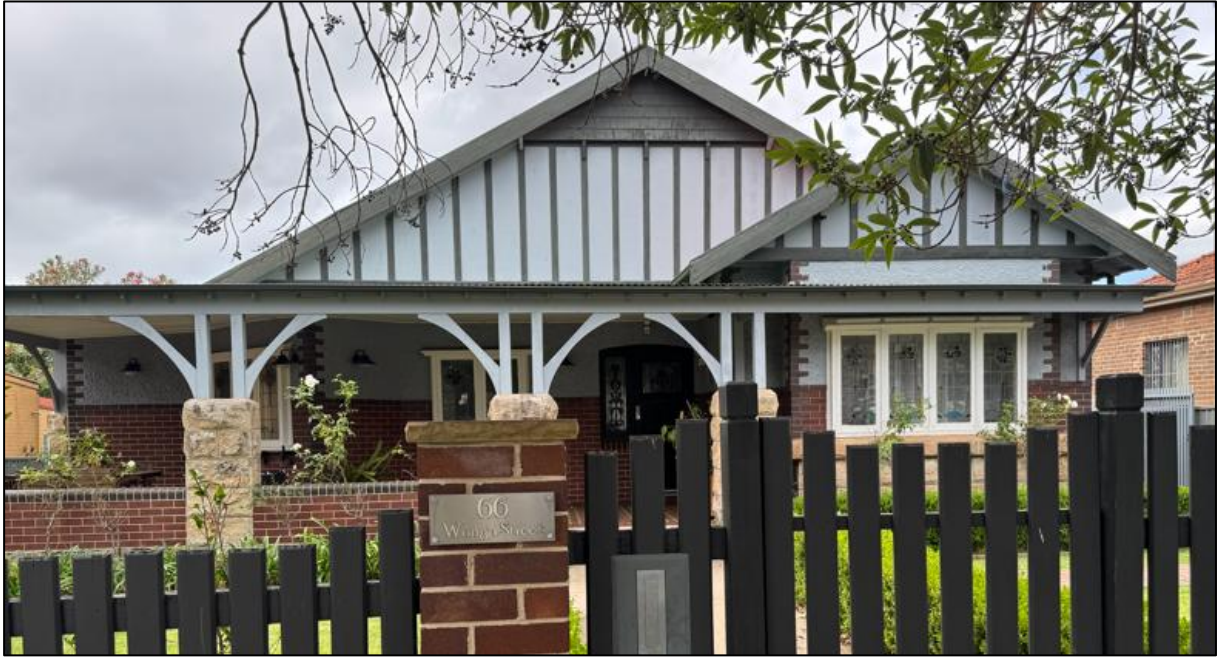
Figure 79: Front elevation of 66 Wonga Street.
