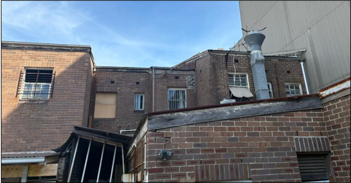
Figure 32: View of rear façade of No. 341-347 Beamish Street.
