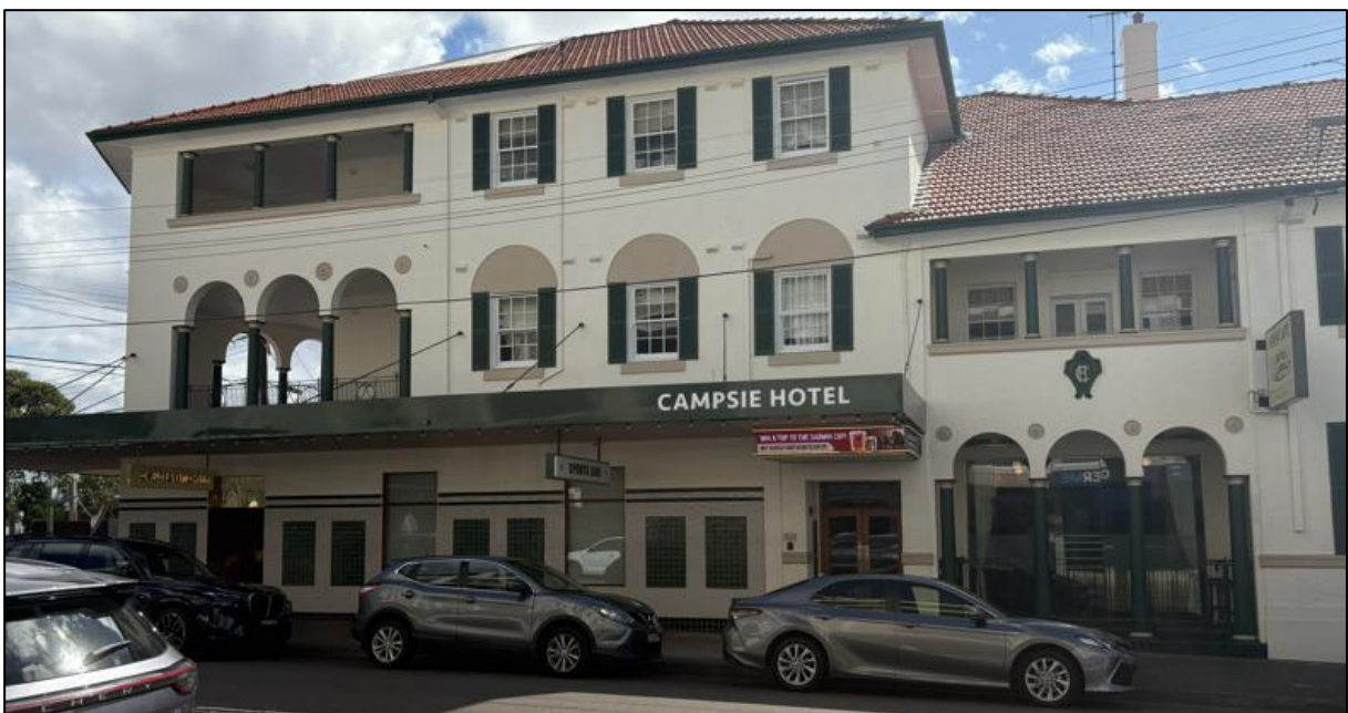
Figure 19: Hill Street façade of the Campsie Hotel.
