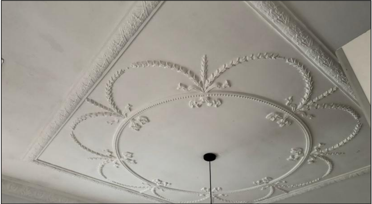
Figure 83: View of the plaster decorative ceiling and cornice within front bedroom.
