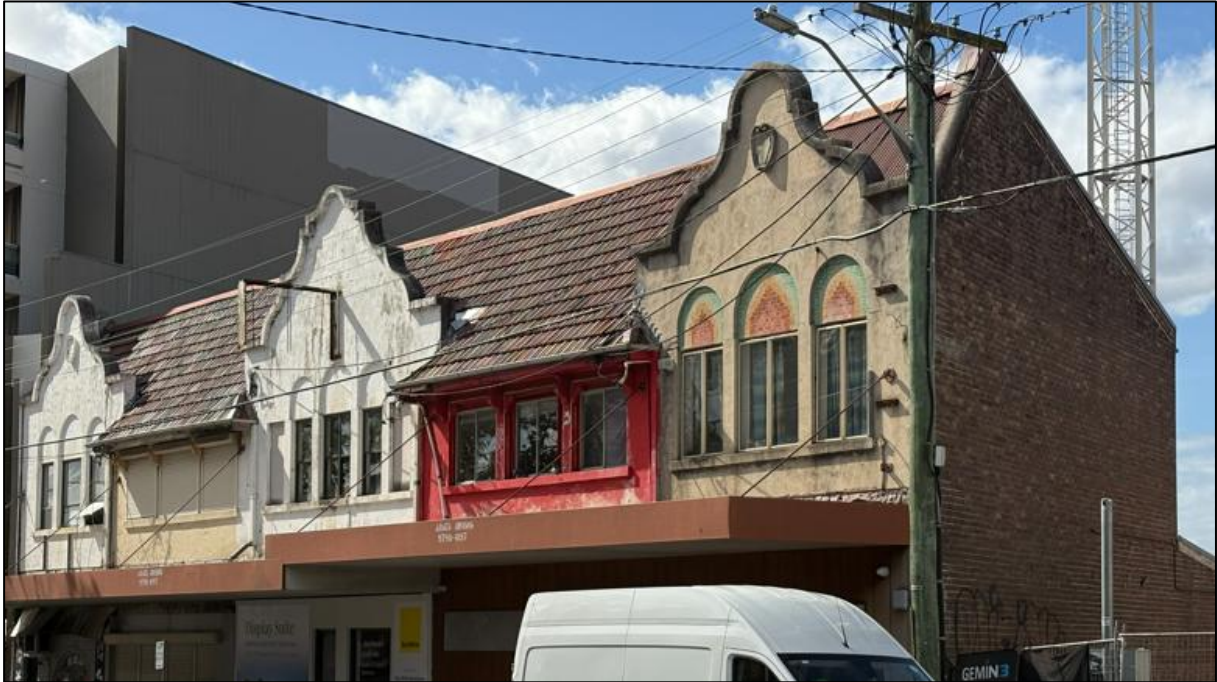
Figure 30: View of the front and southern (side) elevations of the building.
